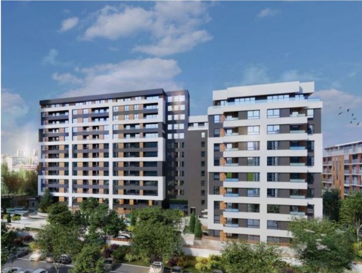
Wellport (Photo: CBS International)
